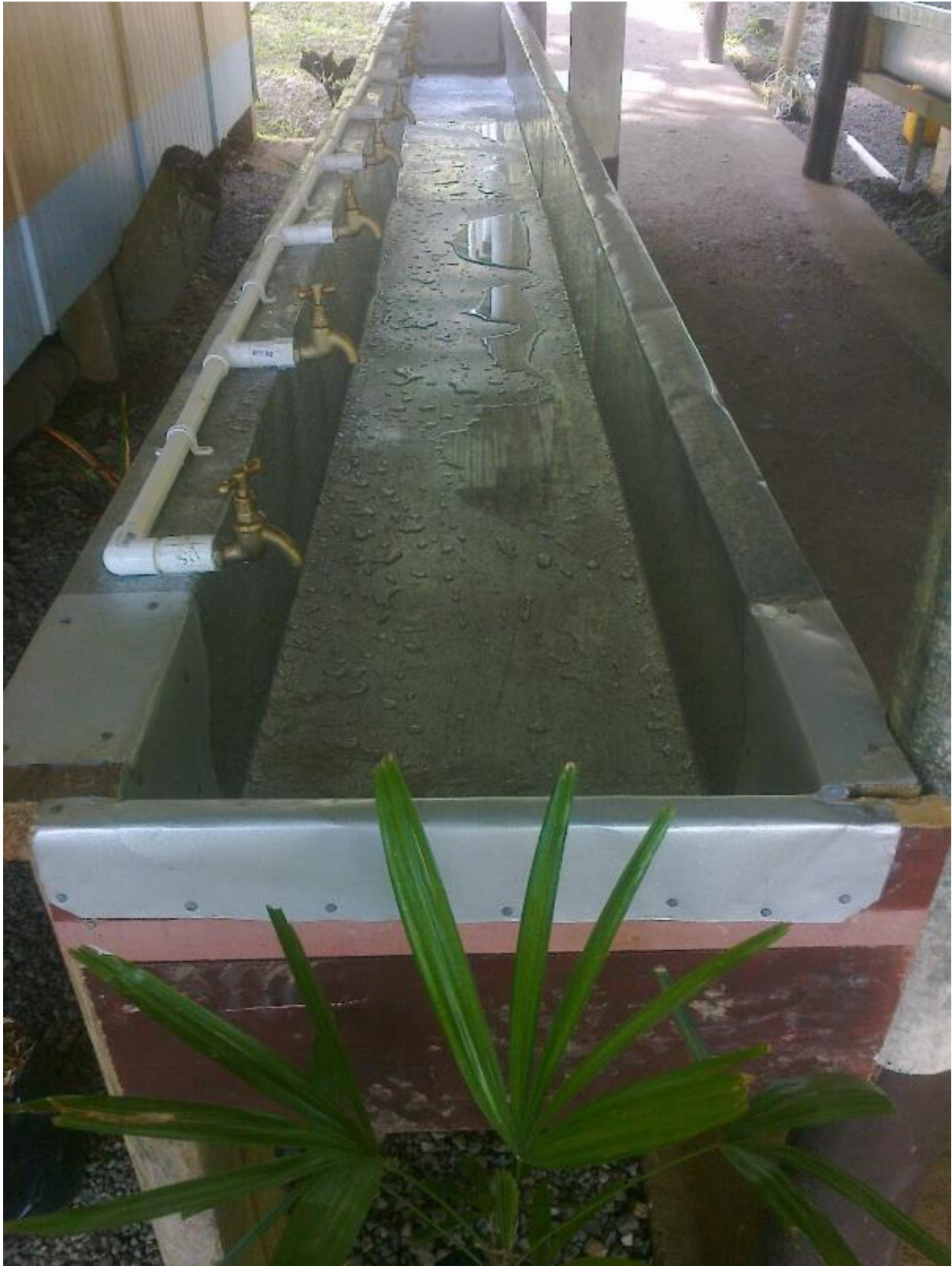
Image 5: Handwashing infrastructure – impact of three star project
